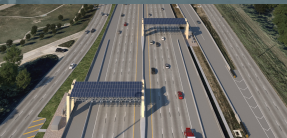
Sam Houston Tollway East from SH 3 to SH 225 Convert East Toll Plaza to Ultimate AET PS&E Package 2, Harris County, TX
