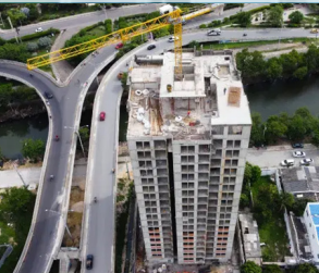
Kaua Building, 110,000 SF, 18 floor residential building, Cartagena, Colombia
