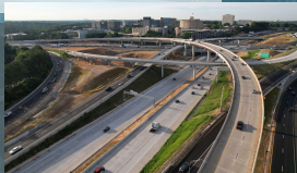
I-285 and SH-400 Interchange Reconstruction, Atlanta, GA
