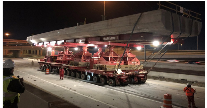
SH 114 Signature Bridge, Irving, TX: Accelerated Bridge Construction
